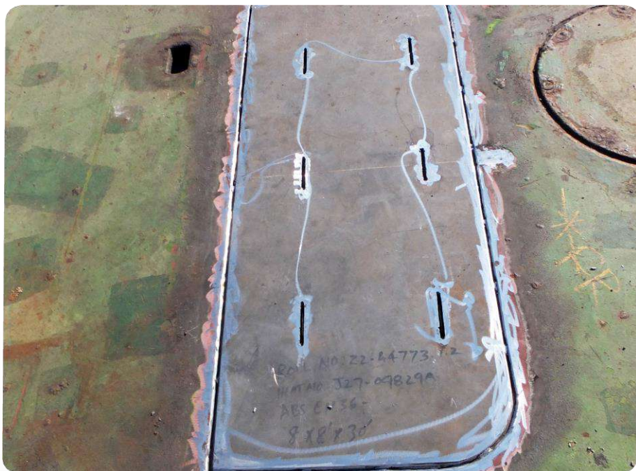
Reinstating works for heavy load transport vessel
