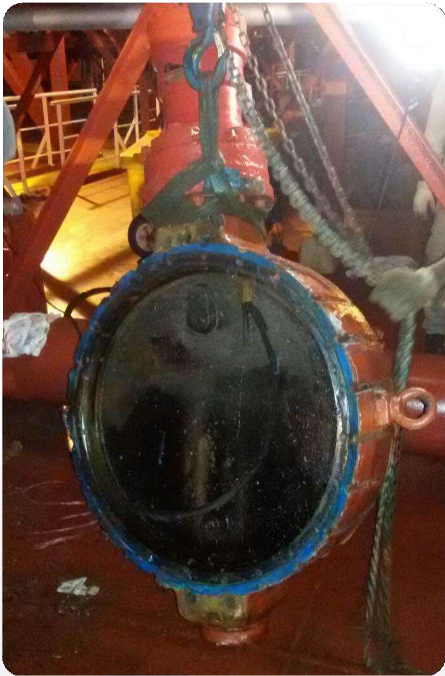
Valve removal & overhauling of PV valve , safety Valves , Butterfly & gate valve
